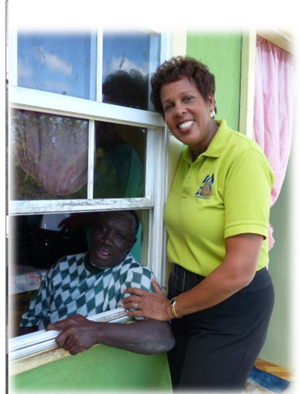
Belfield Hurdle enjoys the fresh St. John air passing through his newly repaired home while chatting with President of the Rotary Club of Barbados, Brenda Pope, during an official presentation ceremony for the club's House Repair Project.
