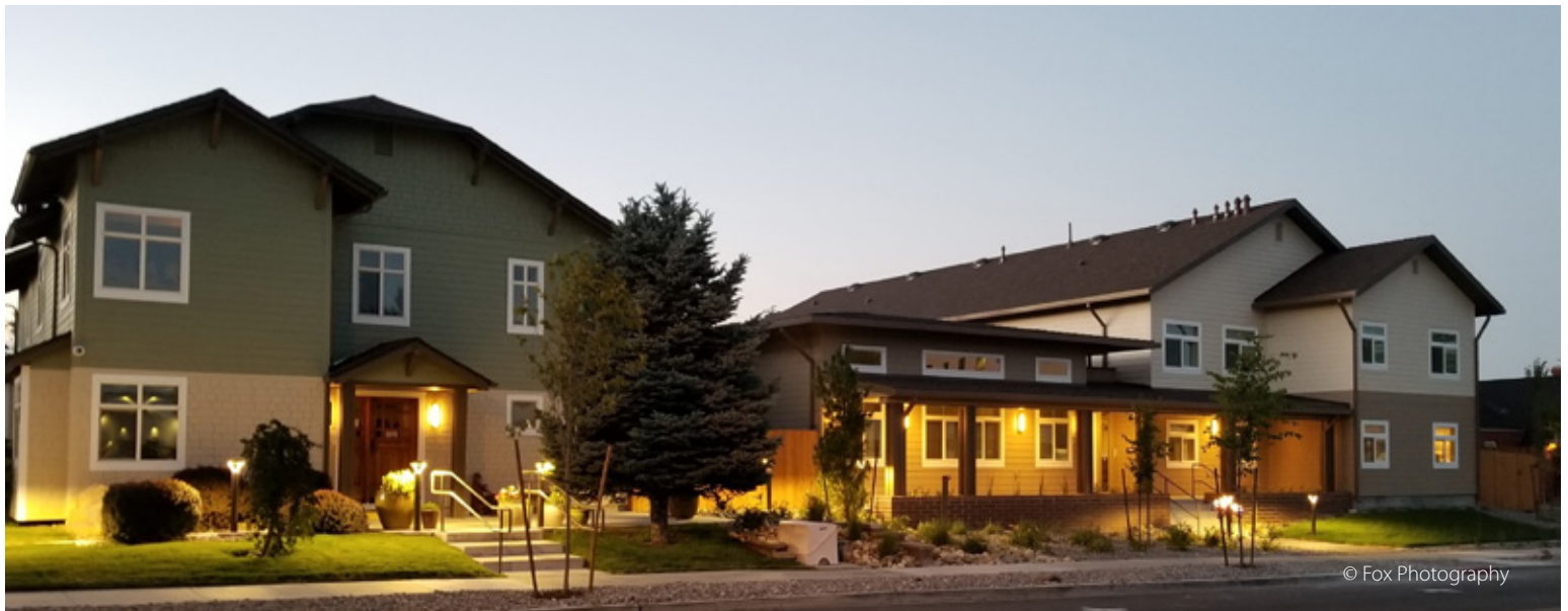
The old and new: the Veterans Guest House expansion is on the right, connected to the existing house on left. (the night time shot)
