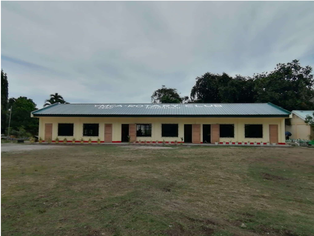
The 3 classrooms as it looks today.
