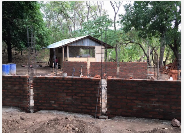
New school building in progress in Piedra de Agua
