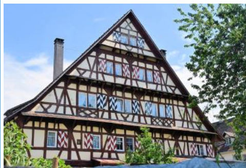
Built in 1661, Bregenz's old town hall (altes rathaus) is a private residence now.
