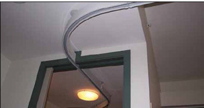
Roof mounted self drive rail system
