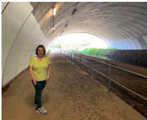
Walking in tunnel under the M2
