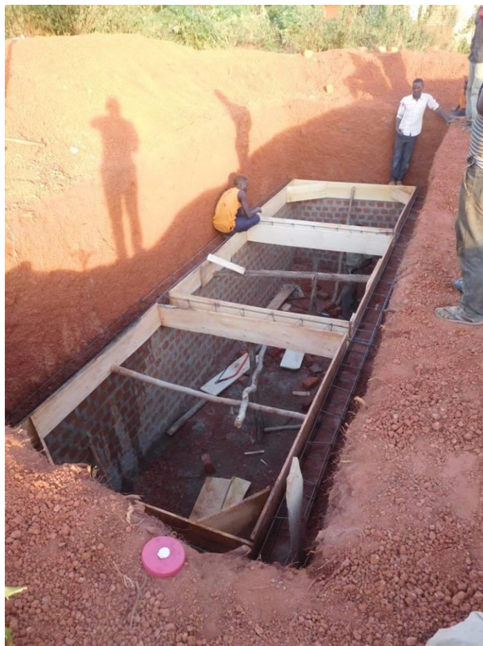
Excavations for the toilets
