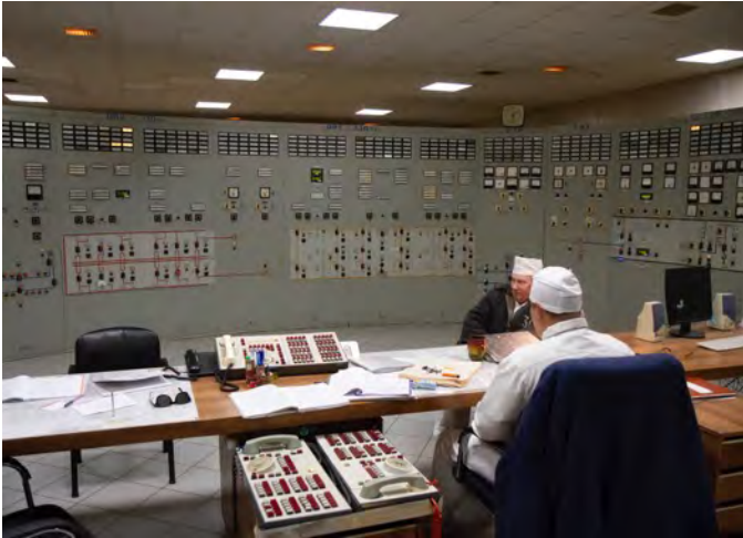
The switchyard control room still controls the electric grid for parts of Ukraine and Belarus.
