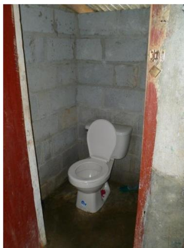
**Installation in the Merendón of a pour flush toilet with laundry and shower connected to a soak away septic pit. Toilet flush is done with a small bucket.**
