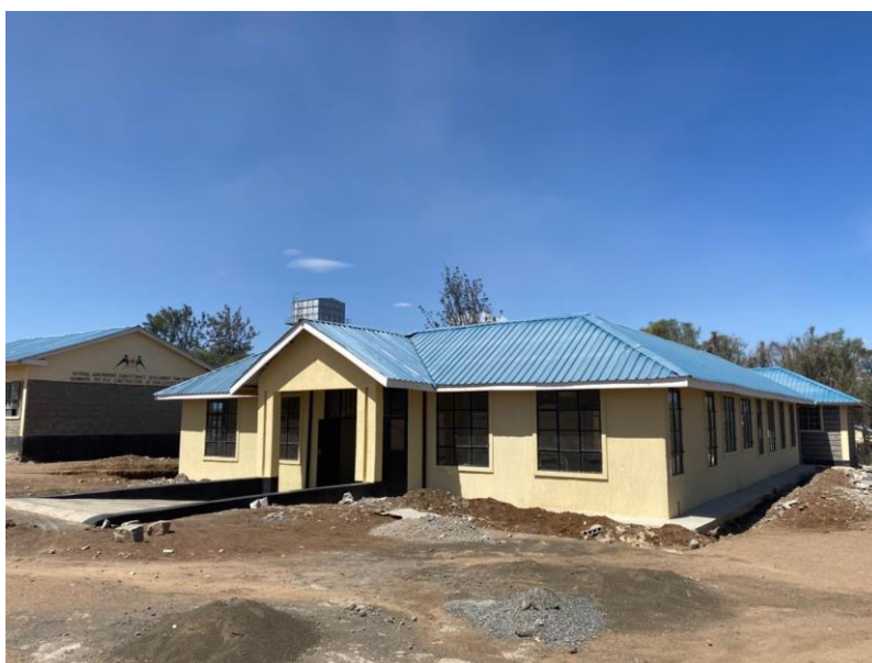
The new school unit with the toilet block at the rear
