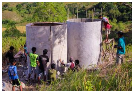
Ferro-cement water tanks
