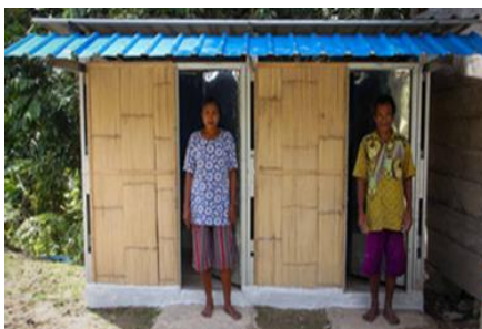
M-F toilets with septic system
