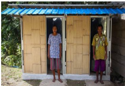
M - F toilets with septic system
