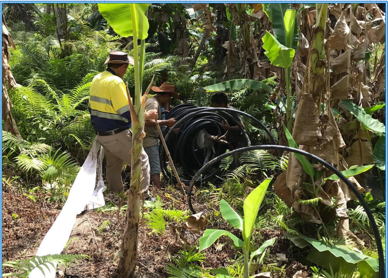
Laying the 4 kilometers of 32 ml poly-pipe
