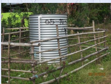
Water tank at Buibela
