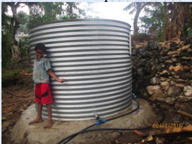
New tanks at Naha'e all connected and overflowing, and stand pipes working
