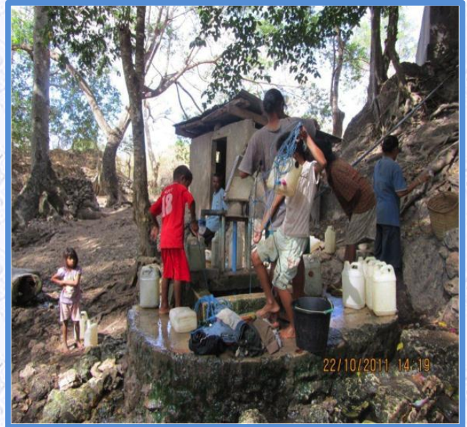
The hand pump was fixed and working again
