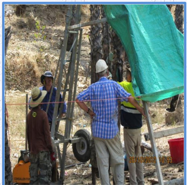
Work commenced on the new bore
