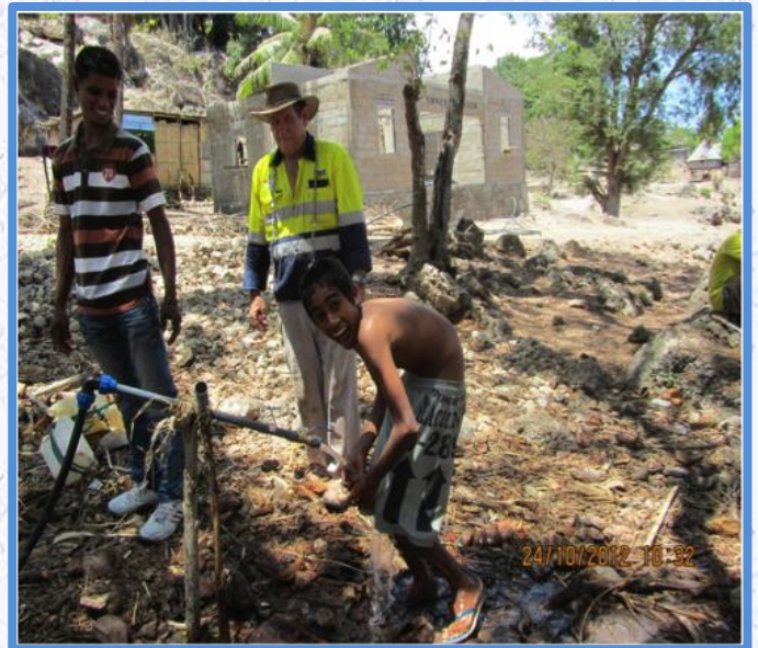
The tap was fitted and the water was flowing
