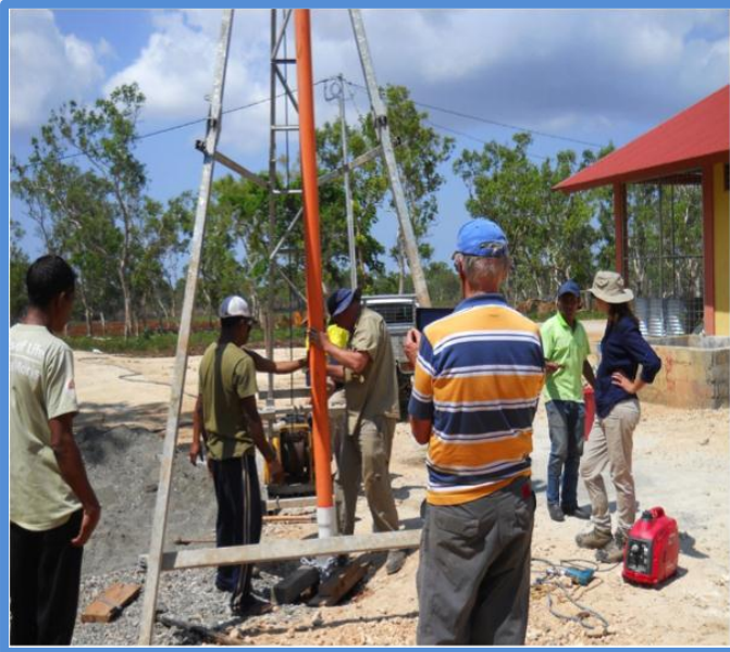
First job was to finish the previous bore
