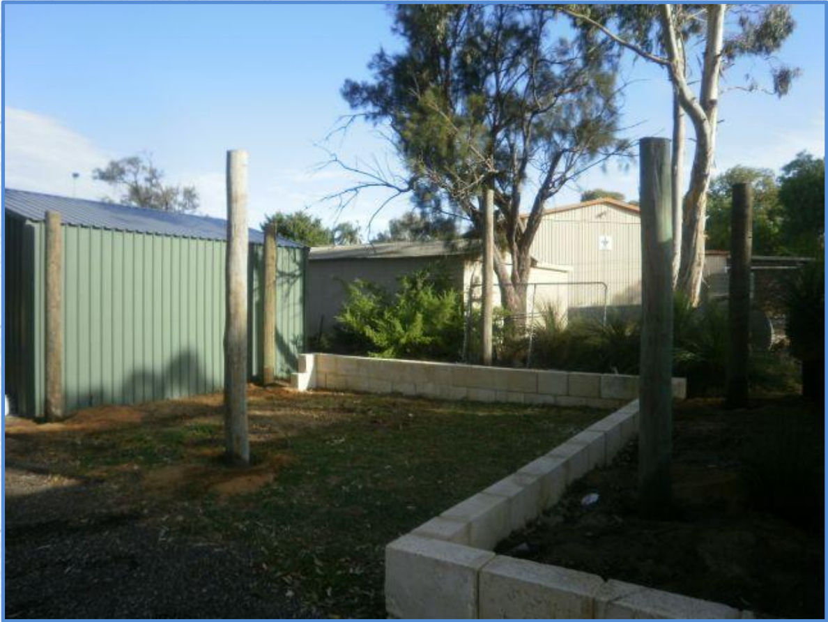
The six poles cemented in and will soon be ready for the shades
