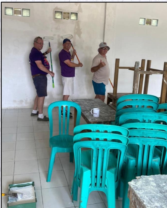
Paint rollers at the 'ready'
