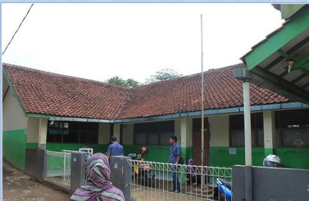
The roof is part of our next project
