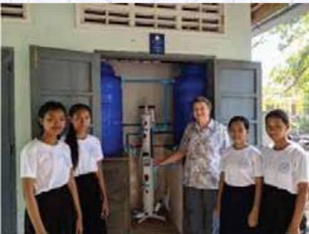
SkyHydrant installation in Cambodia by the Rotary Club of Somerset.
