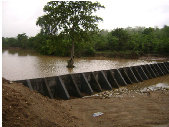
Engineers without Borders water dam project in India
