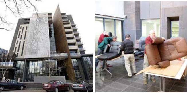
Left: The Elizabeth Street Common Ground facility in Melbourne has provided more than 65 homeless people with affordable housing. Right: Members of the Rotary Club of Melbourne assemble furniture at the facility in 2010. Photo courtesy of the Rotary Club of Melbourne
