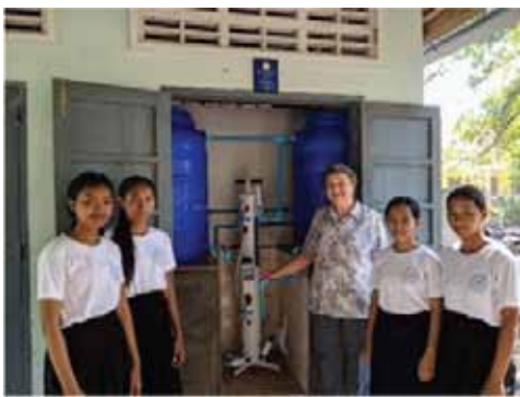
SkyHydrant installation in Cambodia by the Rotary Club of Somerset.
