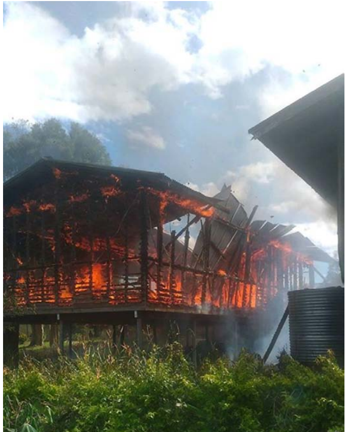
The Nondugl Project Maternity Ward fire
