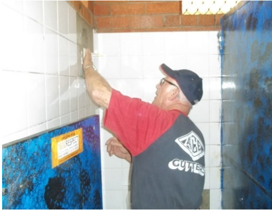
Kevin Sharp replacing tiles on the toilet wall at Rotary Park.
