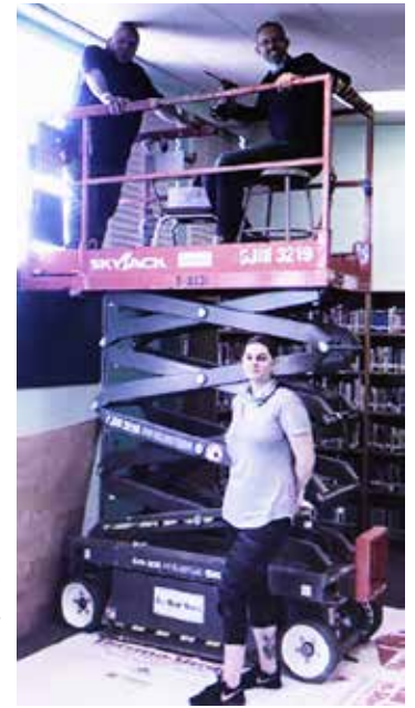
Novato Olive Elementary window shades.
