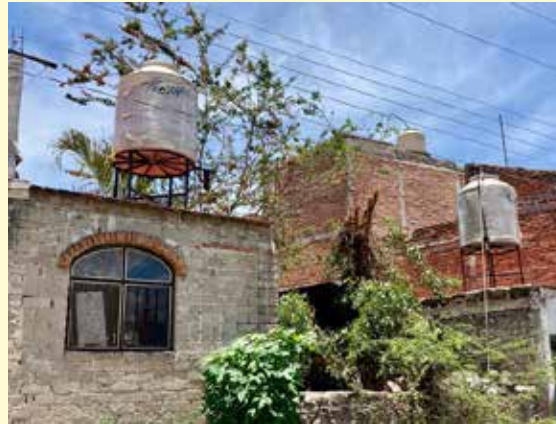
Tinacos and pumps on roofs.
