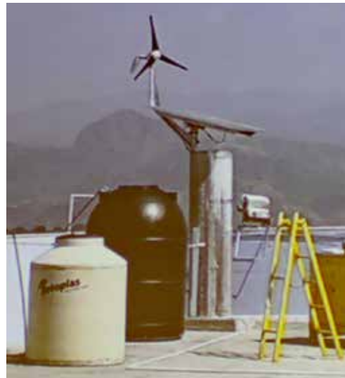
Clean filtered water for drinking and hand washing.
