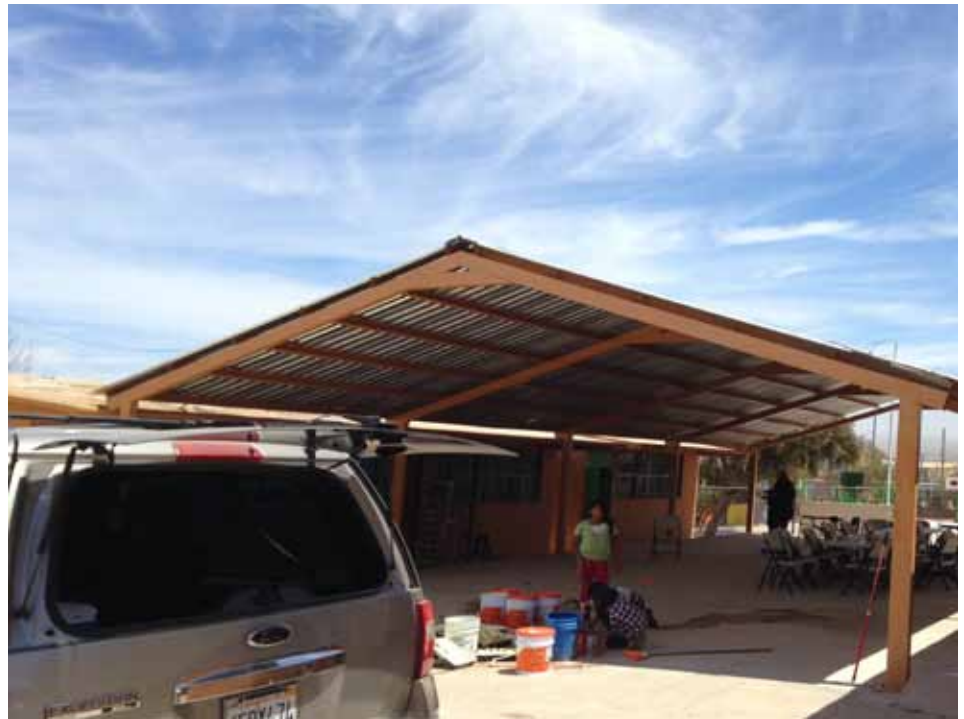
The Old Mission Rotary Foundation funded the design and construction of a a metal shade structure on a concrete pad at the Salvador Diaz School. The structure allows the school children to eat lunch protected from the hot sun of the Baja summer and the rains of the winter.
