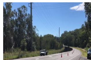
Some of the flood damage still very evident on Friday morning. Top is taken near the Nelson Fish Co-op and the bottom is Nelson Bay Road still flooded 3 days after the rain had stopped
