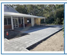
The concrete is cured and ready for the next stage, with brickworks to start this week. Warwick is constructing the bench seats.
