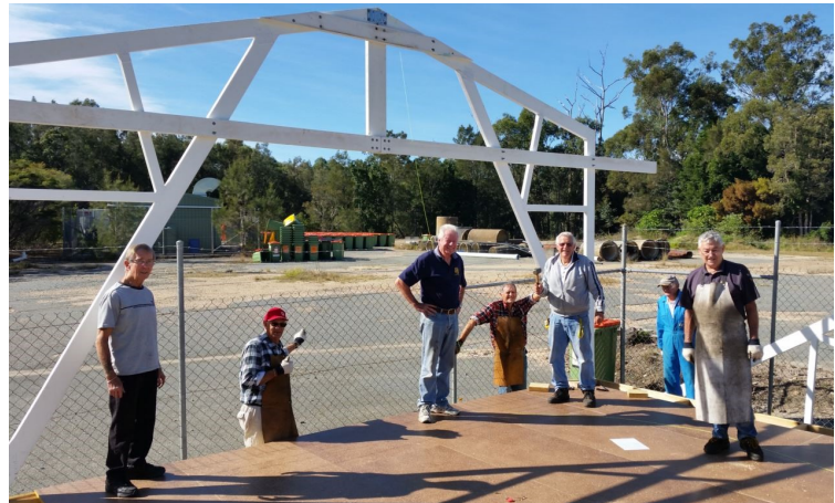
The project is starting to take shape: Pre-sassembly at The Shed
