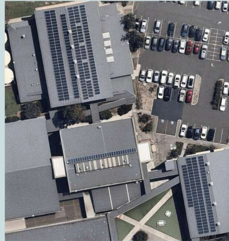
$100,000 of solar installed
