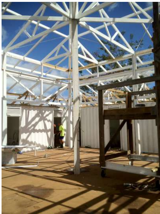
The House of Hope in Apia, Samoa, under Construction. The entire building was pre-manufactured and test assembled at our Project Shed in Arundel, then flat packed into 4 shipping containers, which ultimately became part of the overall structure, with the doors and windows cut out (picture above right). Picture left: view from the inside; the frame is up. Yes! It is cyclone proof too!
