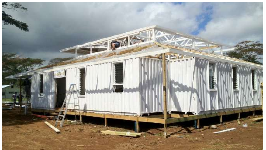
The House of Hope in Apia, Samoa, under Construction. The entire building was pre-manufactured and test assembled at our Project Shed in Arundel, then flat packed into 4 shipping containers, which ultimately became part of the overall structure, with the doors and windows cut out (picture above right). Picture left: view from the inside; the frame is up. Yes! It is cyclone proof too!
