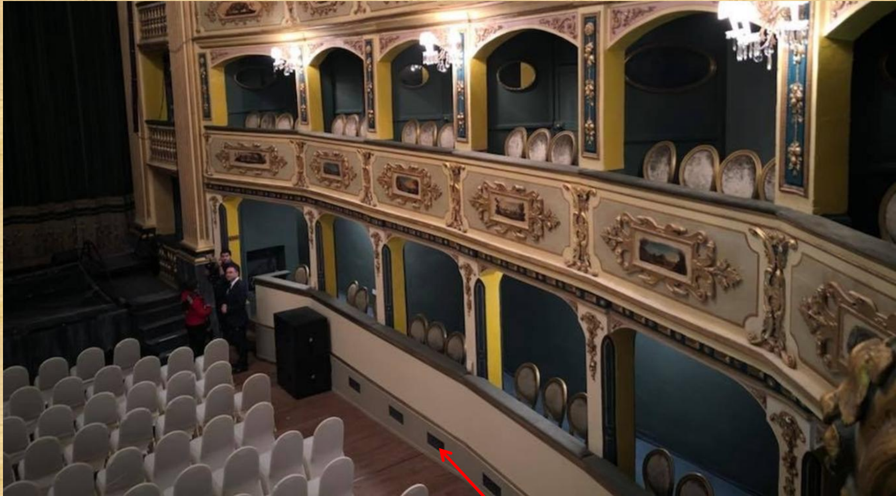
The parterre boxes with the air grilles under the boxes
