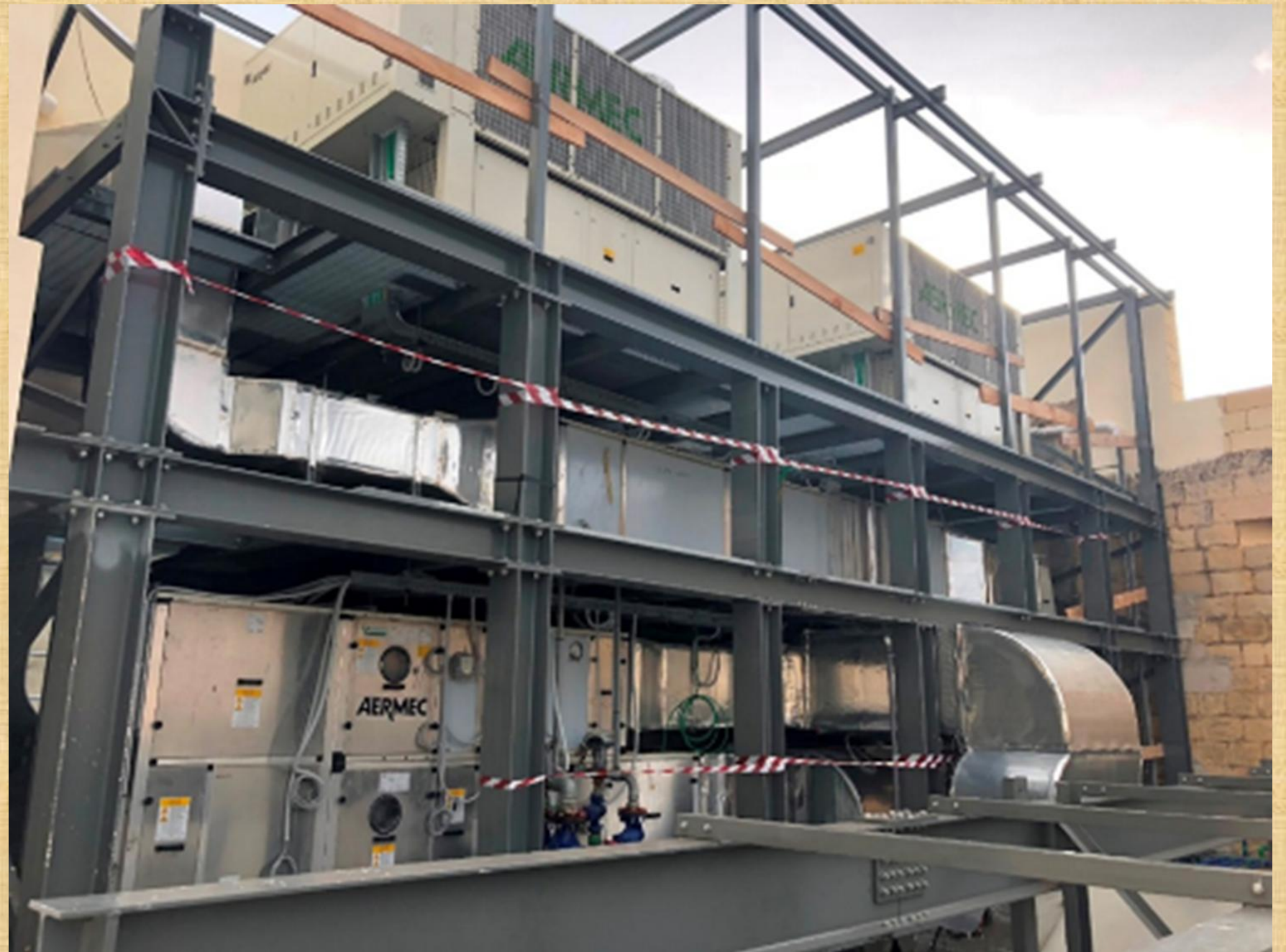
The two-storey structure built to accommodate the machinery
