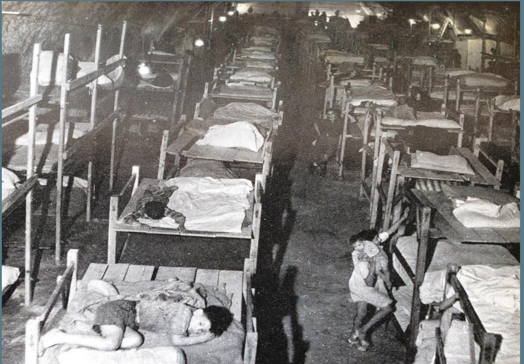
War time shelters in tunnel in the landfront ditch formerly used by the railway
