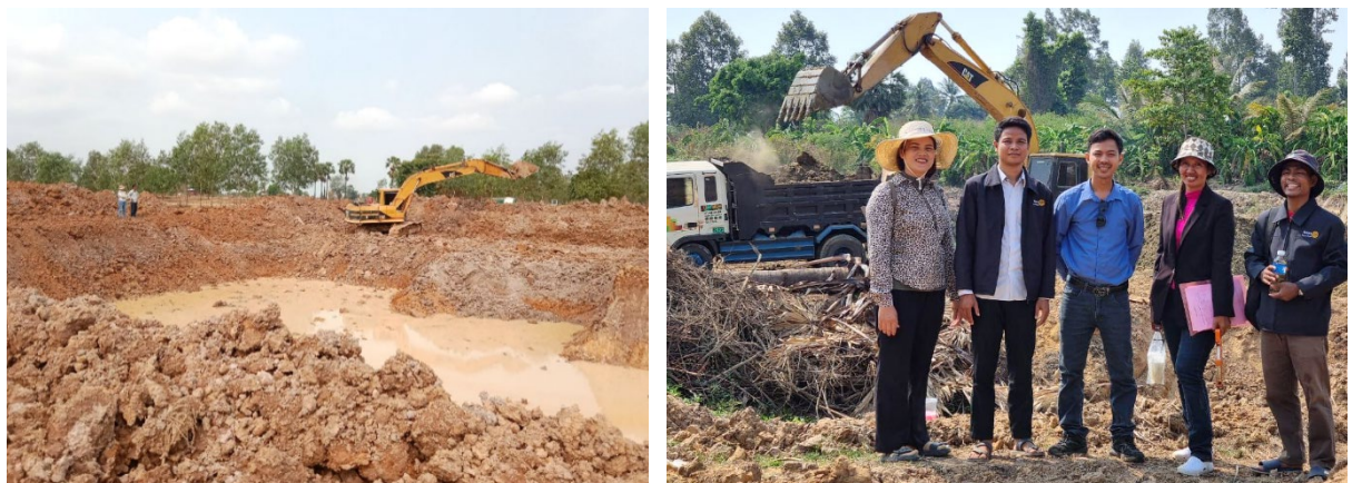
Photos of the procurement committee monitoring the community pond excavation
