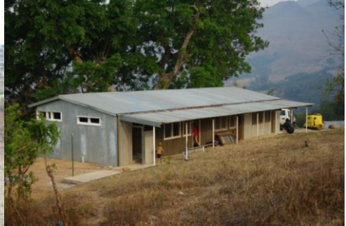
Almost completed new school
