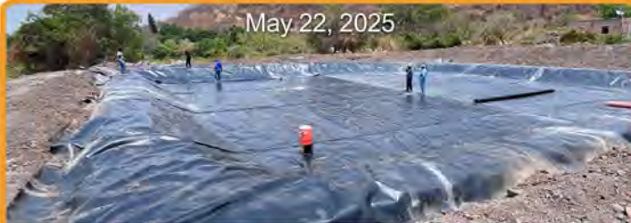
The polyethylene Humedal (pond) liner being installed
