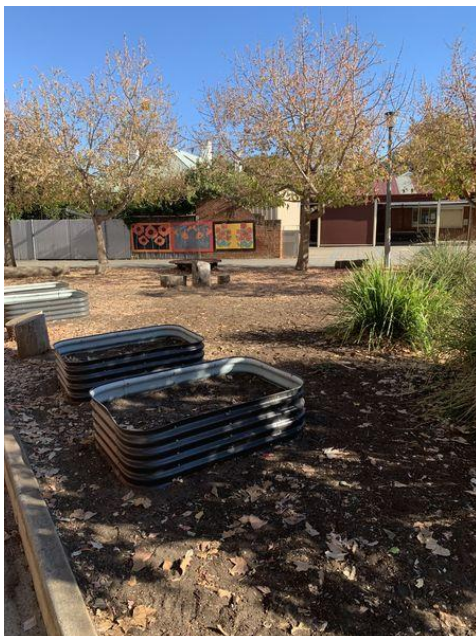
Large area ready for the next stage.
