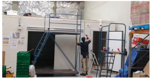
Progress photo showing the new chiller/freezer room under construction
