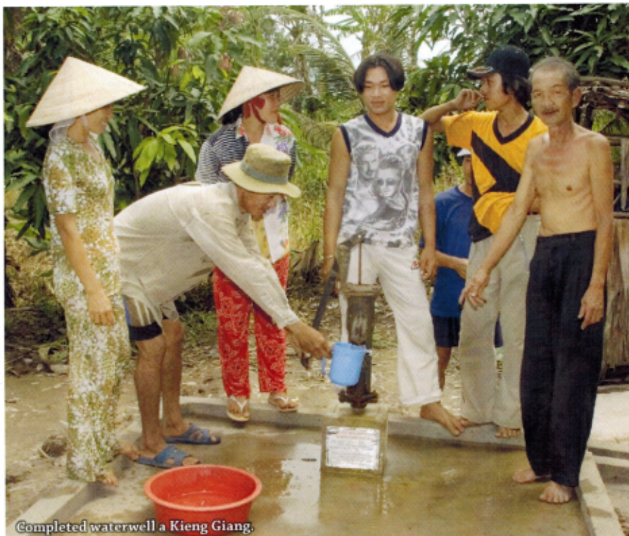
Completed waterwell at Kien Giang.
