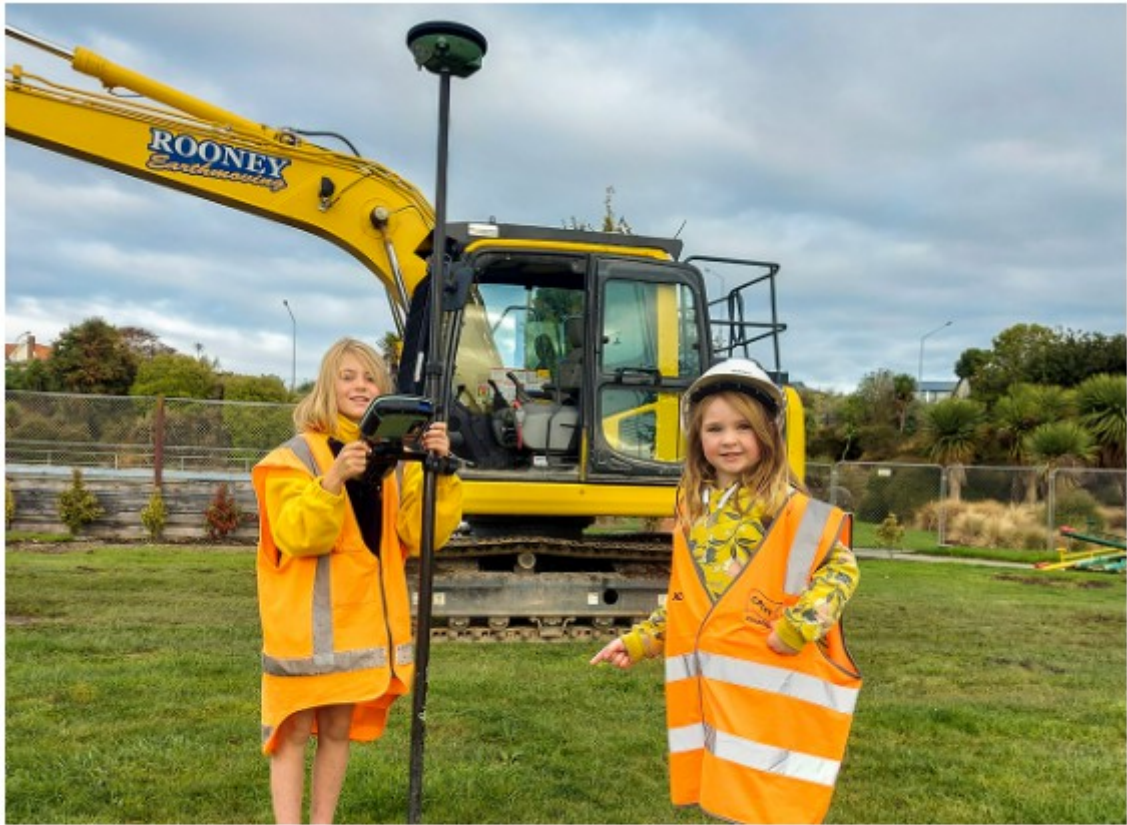
Before the earthworks got underway, sisters, Medinella 8 and Annabelle 4 Fauth, were shown how the Rooney Earthmoving team use GPS to mark out the playground plans on the surface.
