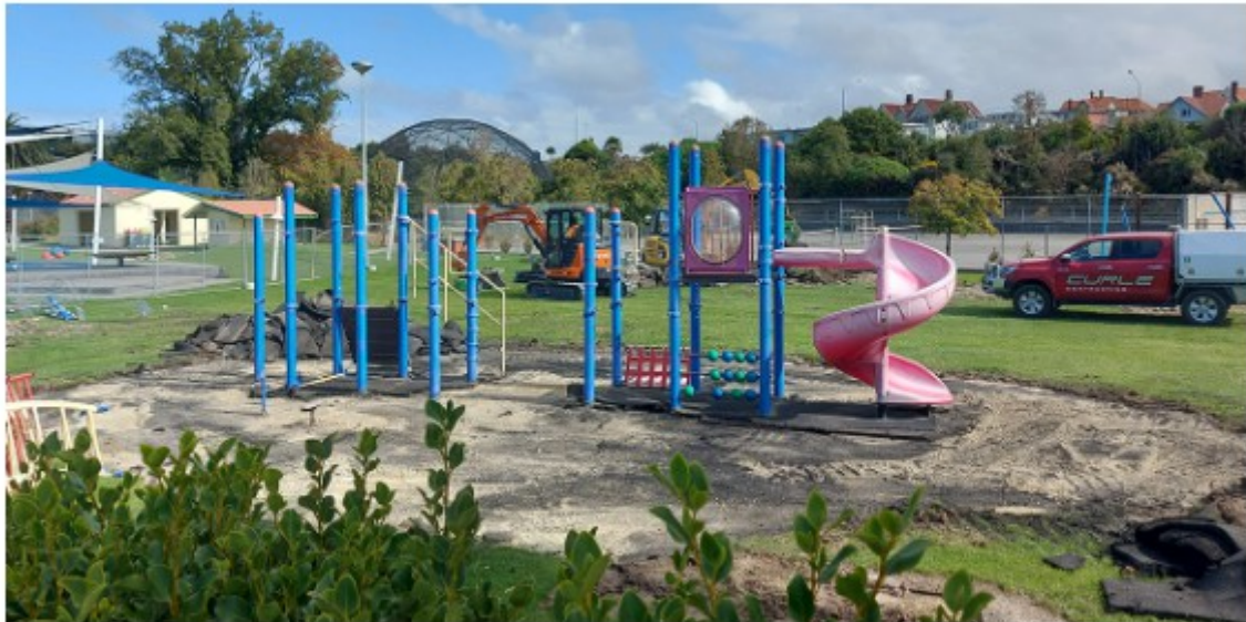
Above: Dismantling equipment to shift off site.
