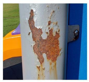
Here is an example of a playground in Timaru, where it looks like powder coating has been applied directly to the black steel. You can see how the paint has bubbled away and the steel is rusting.
