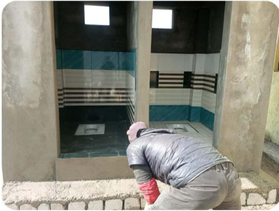
The tiles in the toilet (indoor) have been installed and plastering work is in progress.
