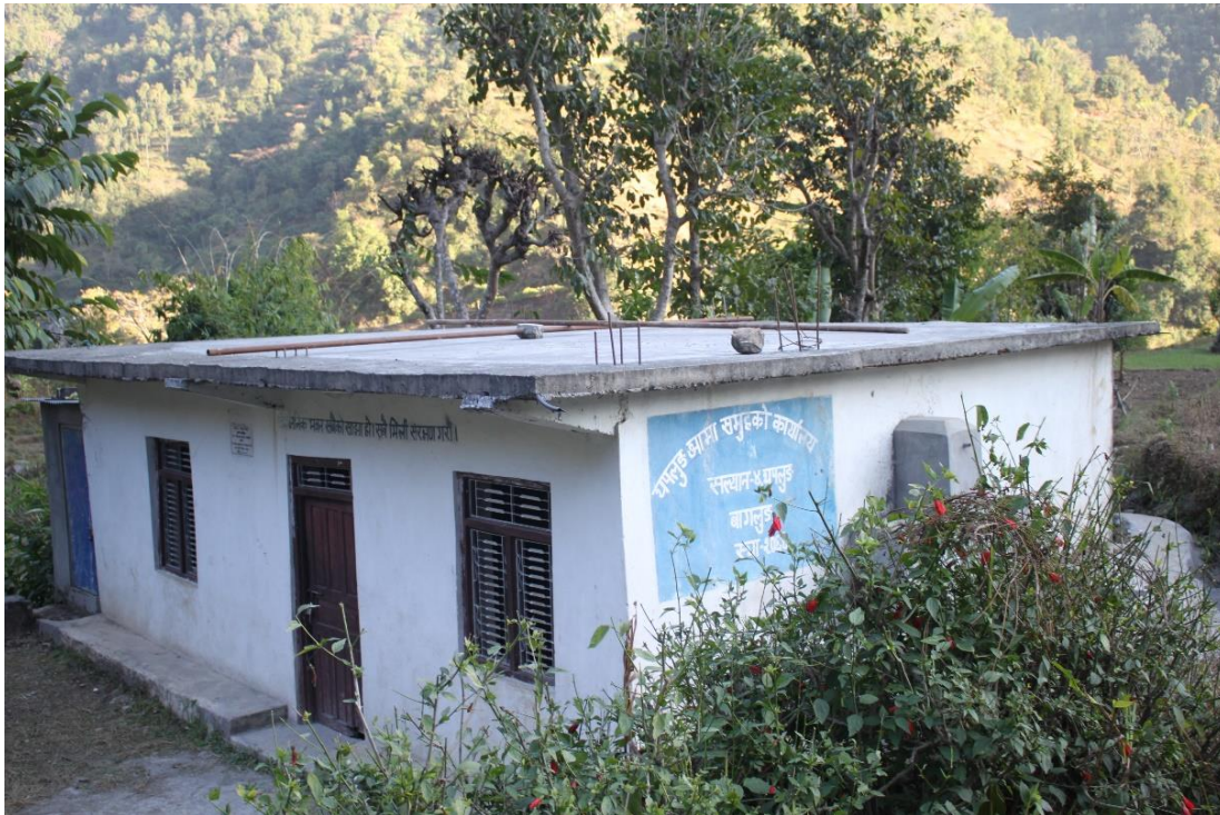
Photo 2: Building before construction of Health Unit
