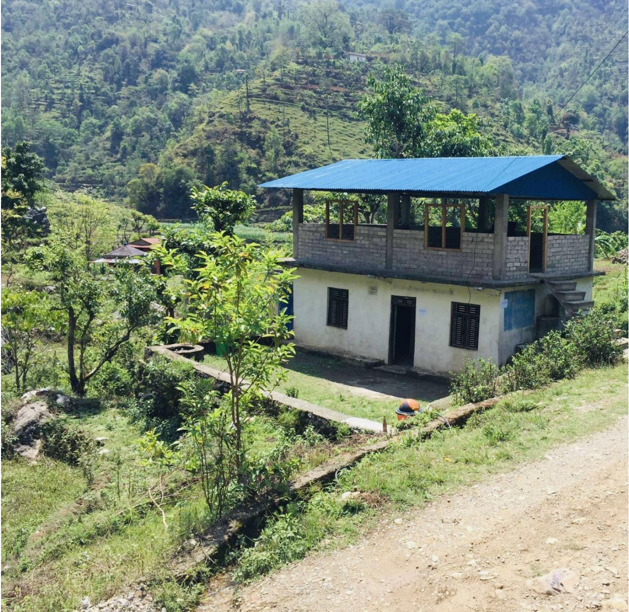
Photo 3: Building under construction with green environment in the background
