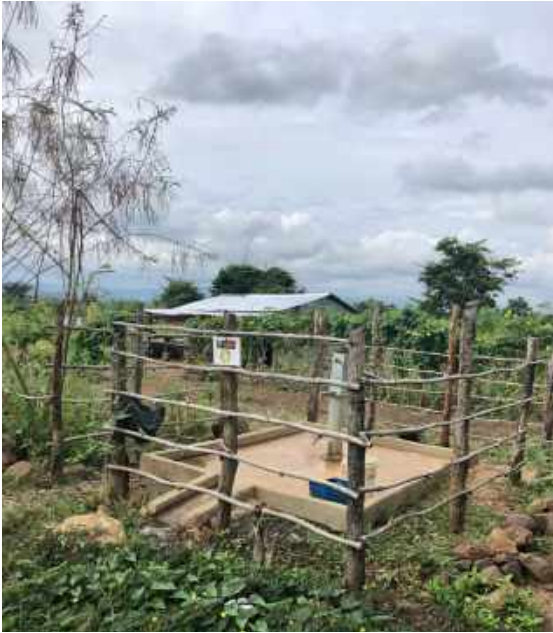
Another village bore and pump – had to drill down 70 meters to hit water
