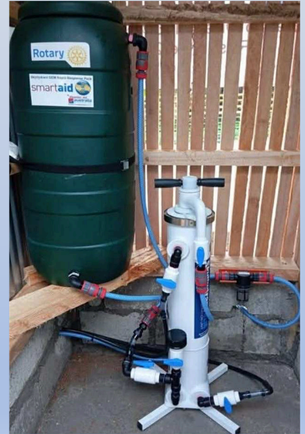
Fixed installation at Barangay Ban-ao, Baganga with Disaster Aid Australia
