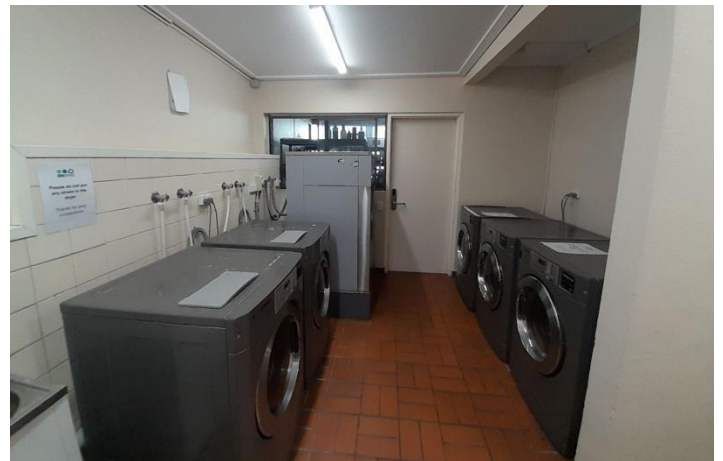
Laundry – extensively cleaned & repainted same colour
