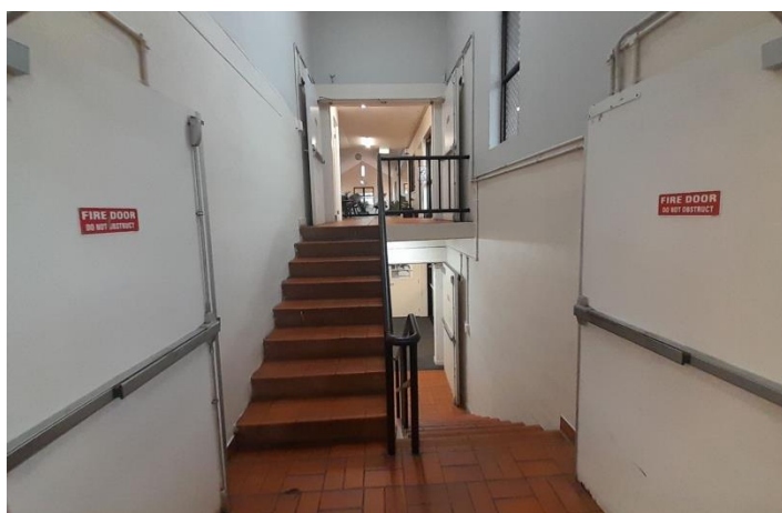
Central stair looking up to top level – the light walls used to be olive green and the handrail was a badly scratched light blue
